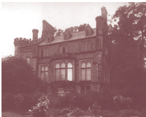
Bolton Hall before it was demolished.
